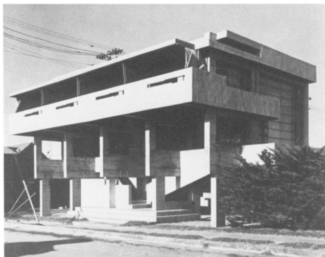
Fig. 3. Schindler, Beach House, street elevation (north elevation), 1926. Photo taken before the wall was built (UCSB-ADC).
